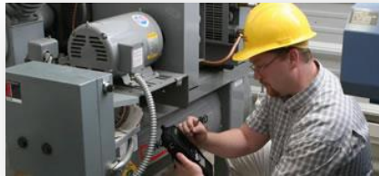
Field Service & Facilities Management
