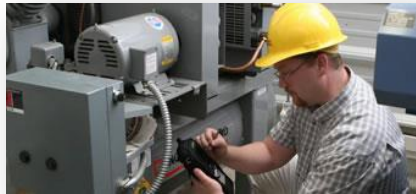
Field Service & Facilities Management
